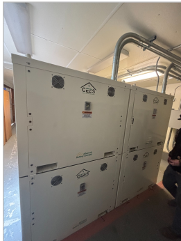
CEES™ units stacked and bolted, direct installation
